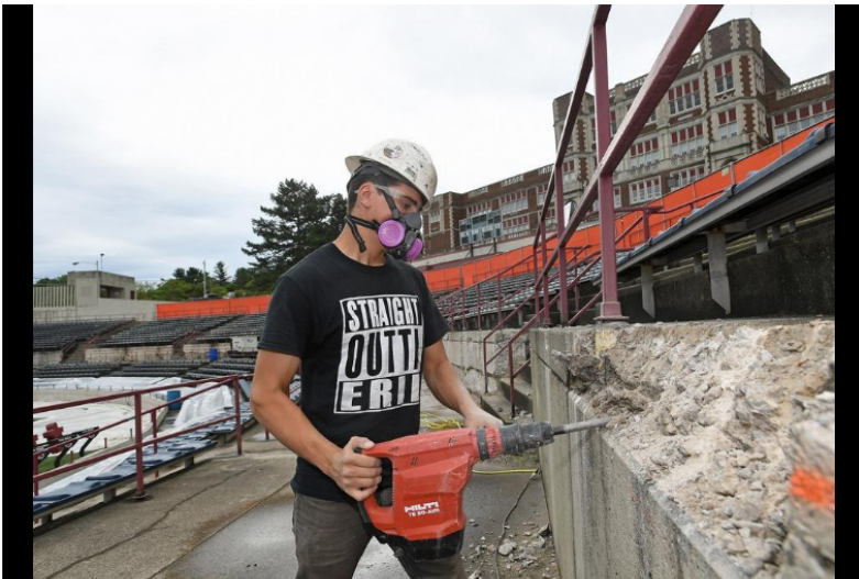
Colton Fleming uses a chipping gun to break away concrete from the walls of Erie Veterans Memorial Stadium on Monday. Fleming, 22, works for Carl Walker Construction of Pittsburgh, which is doing much of the stadium's renovation work. [CHRISTOPHER MILLETTE/ERIE TIMES-NEWS]
